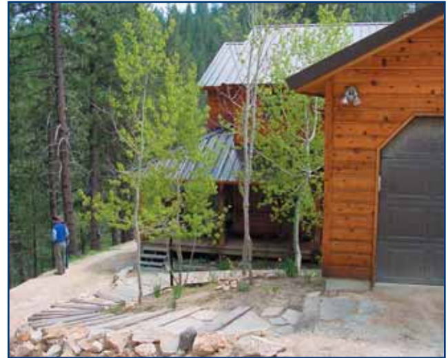
The pre-fire activities implemented by this homeowner include a maintained landscape, use of fire resistant plants, reduced vegetation around the home, and fire resistant roofing materials.
